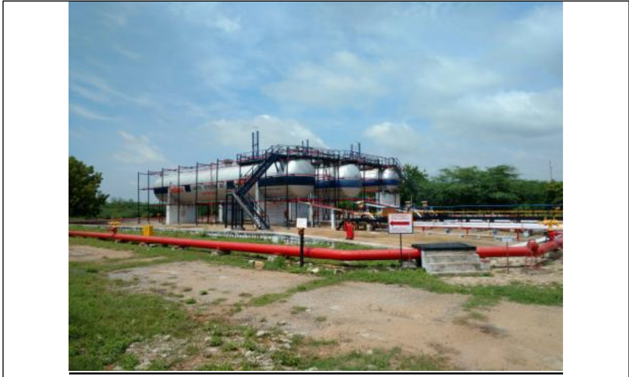
Figure 2.1: Photographs of Existing Tiruchirapalli Bottling Plant
